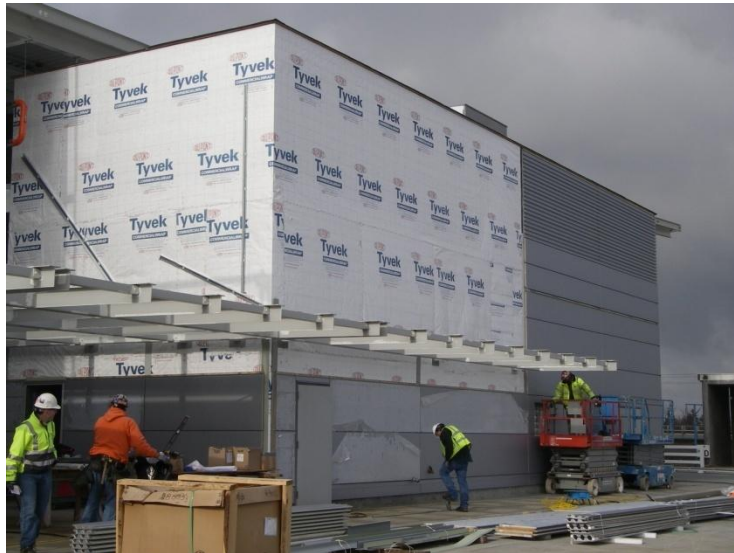
NW Support Building Cladding Installation
