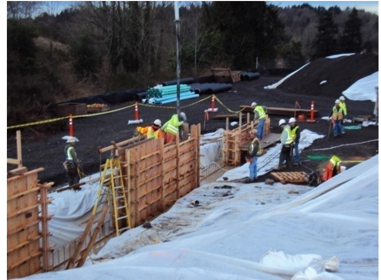
BMF South Ramp Retaining Wall Placement
