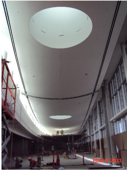
CSB Vaulted Ceiling Installation Progress
