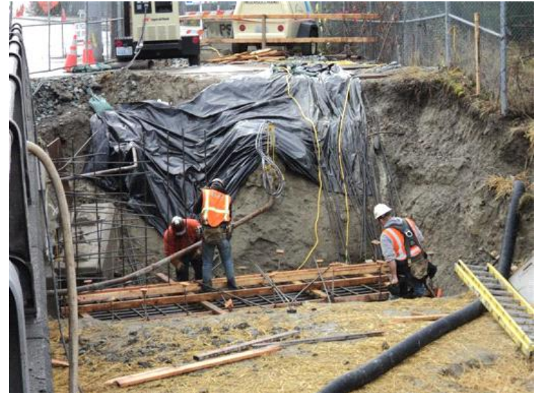
ORI Forming and tying rebar at Abutment 1
